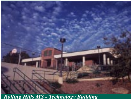
Rolling Hills MS - Technology Building
