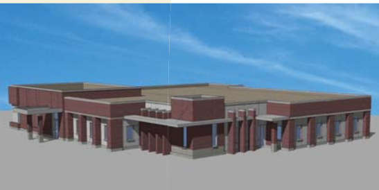
CRC Police, Printing and Nurse Facility - Sacramento, CA
