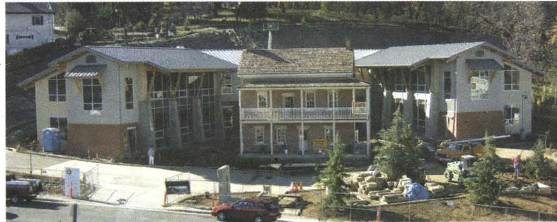
The 147-year-old Fausel House, Placerville's oldest residence, was preserved and restored in Anova Architects' new office complex. The entire project received LEED gold certification.
